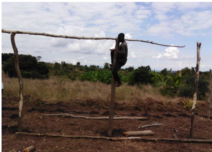
A church member setting a pole
