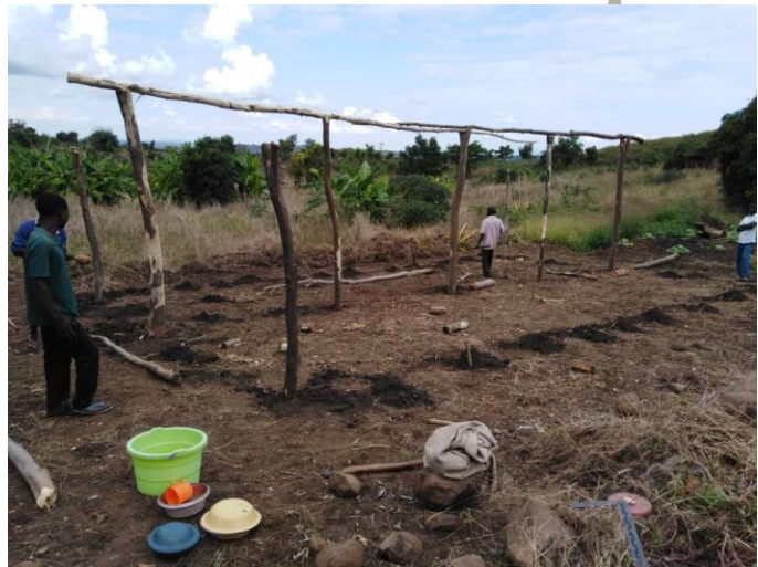
The church being built
